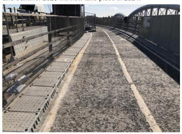
The south cantilever was closed to pedestrians, cyclists and mobility scooters at the end of September to undertake the first phase of the works. This will then enable the cantilever to be used by all other traffic when the works move onto the main deck of the bridge, maintaining the four traffic lanes that the bridge usually operates to reduce potential disruption and delays for the remainder of the scheme.
